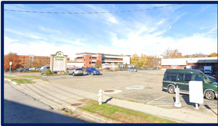
The Gateway Center on Water Street, set to benefit from the Minnow Brook Culvert Rehabilitation Project, ensuring improved access to the vital services housed within the building.
