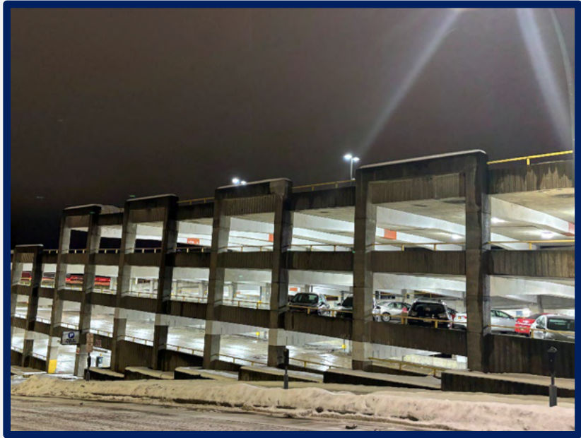
A side view of the Spring Street Ramp at night.
