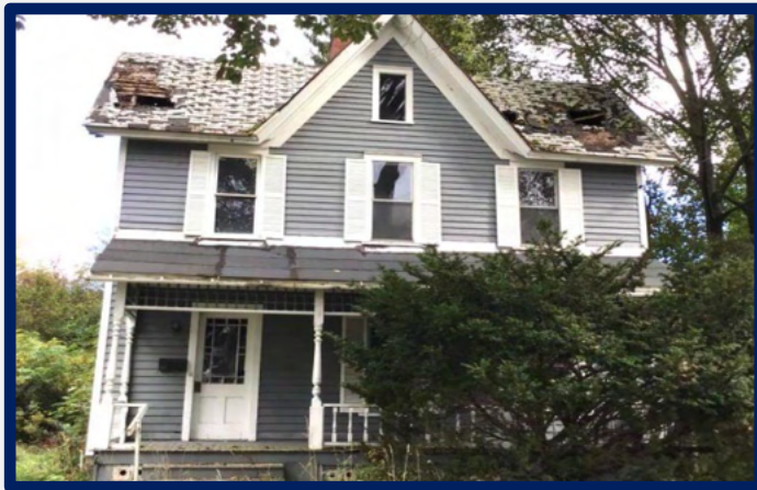
Jamestown's 810 Spring Street was successfully demolished this past spring.
