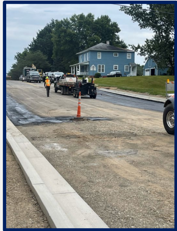
Baker Street captured before the new paving was completed.
