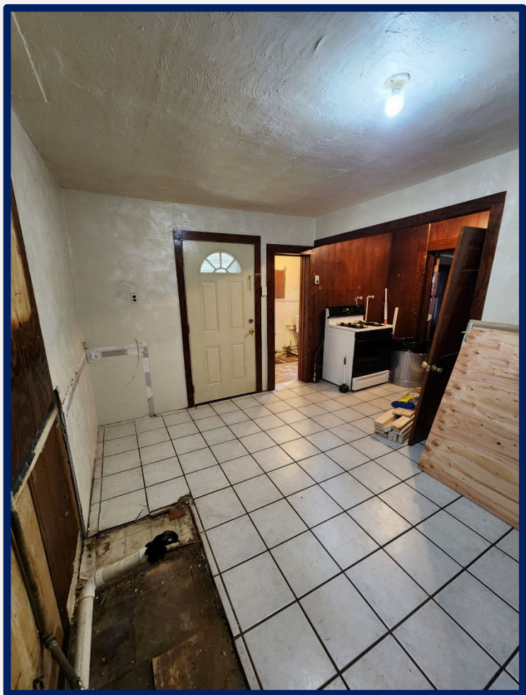
Before Photo: A HOME-ARP – Rental Rehab home undergoing demolition and repairs.
