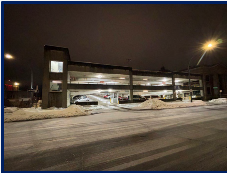
The Spring Street Ramp entrance shines bright at night, showcasing the new cameras and enhanced lighting that have significantly improved safety and security.
