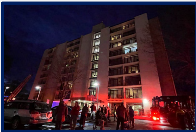
March 11, 2024 – A tragic fire occurred on the 7 th Floor of the High-Rise Senior Apartments on West 5 th Street, resulting in the loss of one resident's life.
