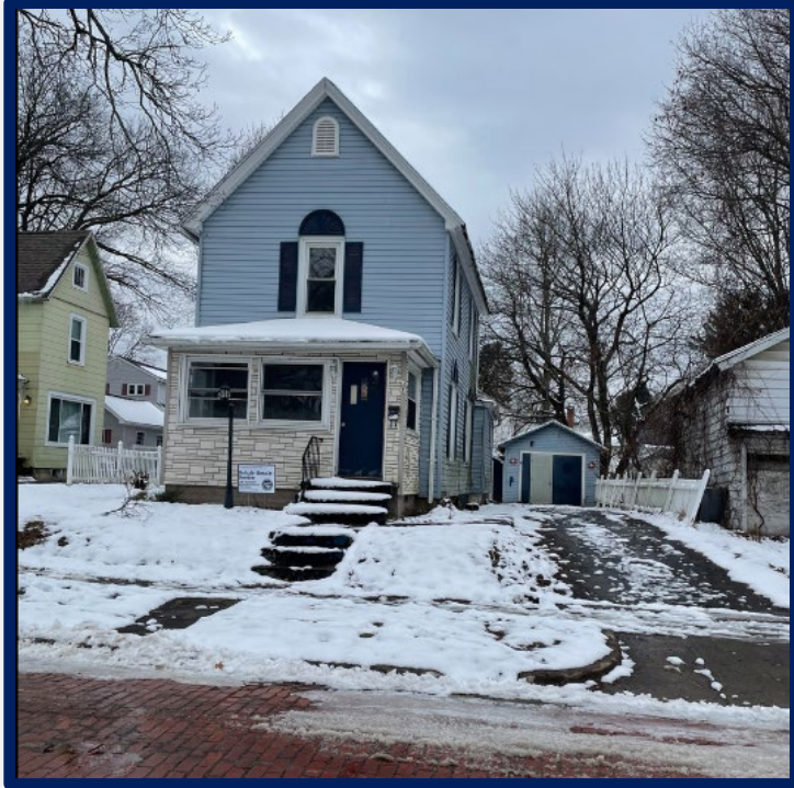
A 19A program property at 49 Utica Street, featuring a city sign highlighting its inclusion in the 19A program and its readiness for rehabilitation.
