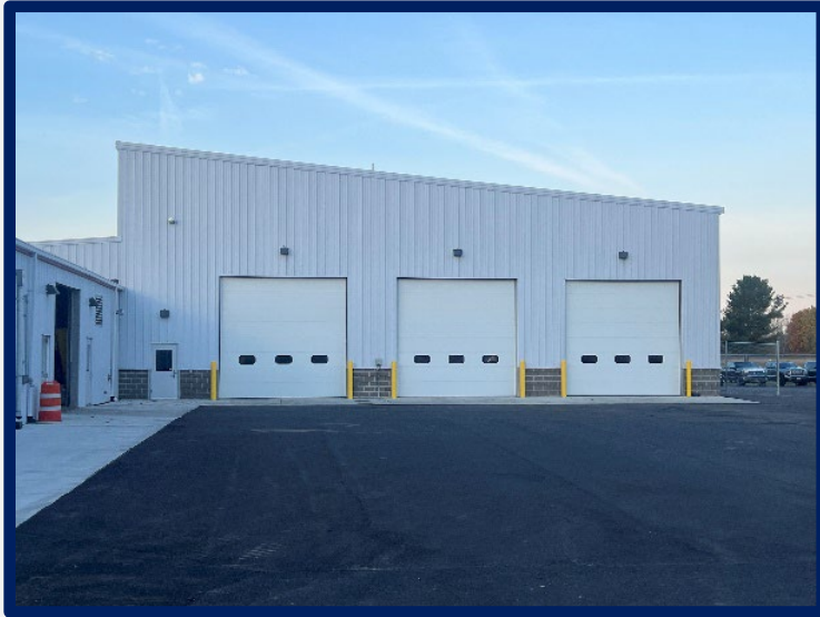
The new Fleet Maintenance Building on Washington Street is now complete and fully operational, ready to service the city's fleet needs.
